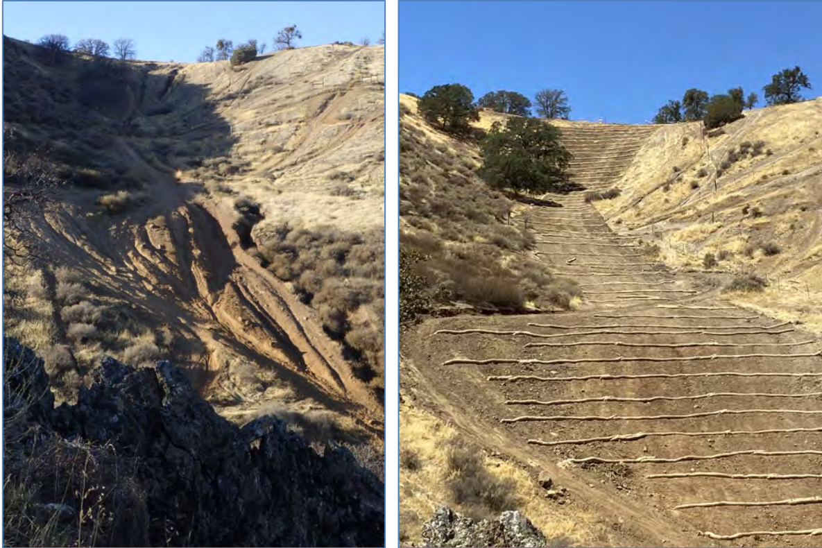
Figure 2-20: Kiln West Hillside Before (Left) and After (Right) Rehabilitation Efforts
