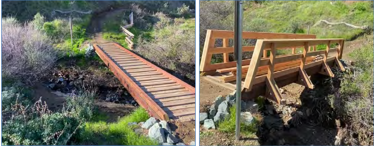
Figure 2-19: Bunkhouse Bridge with Railing (Left) and without Railing (Right)
