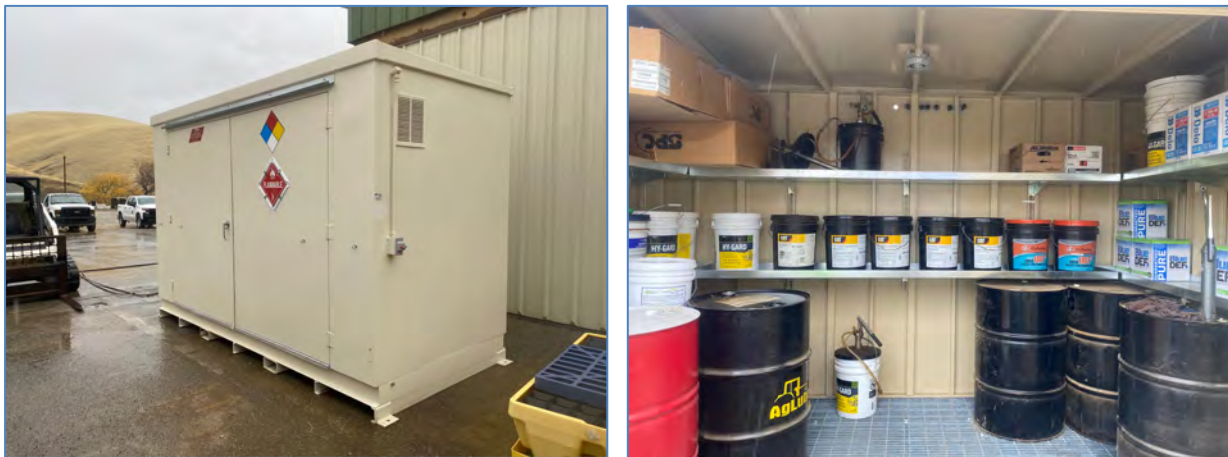
Figure 2-12: New Oil Containment System at the Carnegie Maintenance Shop
